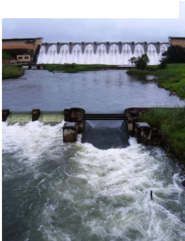
Overflow of Midmar Dam flowing into the Umgeni River
